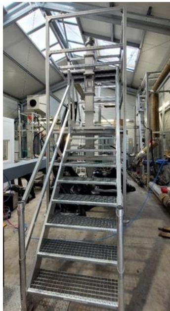
Figure 4: Structure and stairs
